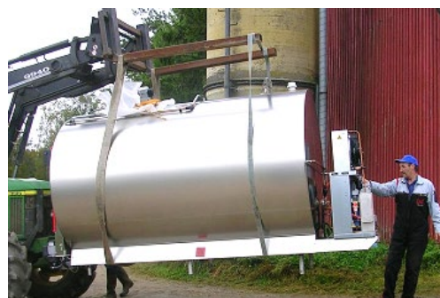
Picture 5. When using lifting belts, it is important to secure the belts at both the fork and the tank. Note the distance between the front loaders and the tank – check if the door opening is high enough.
